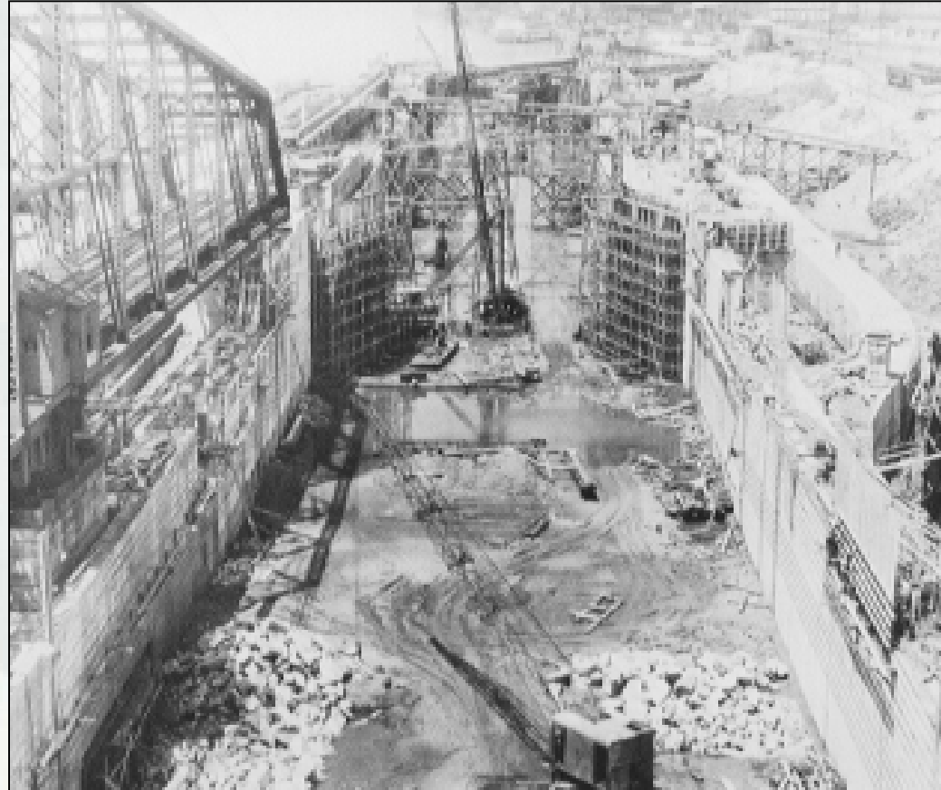
Lock and Dam #26 Under Construction
