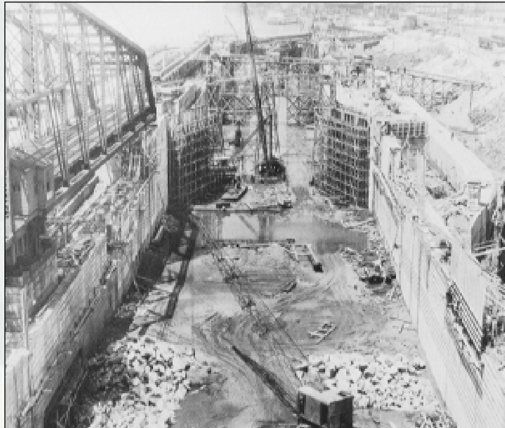
Lock and Dam #26 Under Construction
